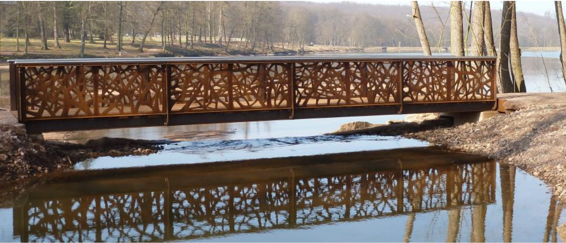
Corten steel cladding with the texture of ornamental branches
