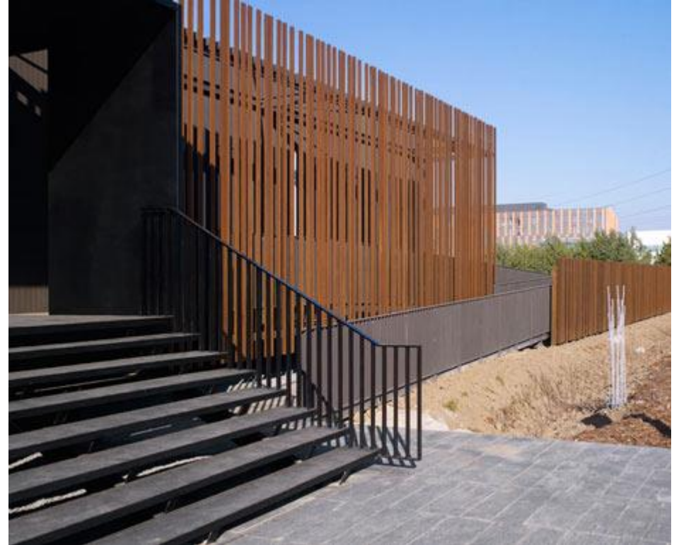
Example of a building cover from irregular sized beams (here: Corten)
