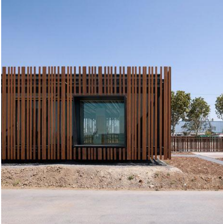
Example of a building cover from irregular sized beams (here: Corten)
