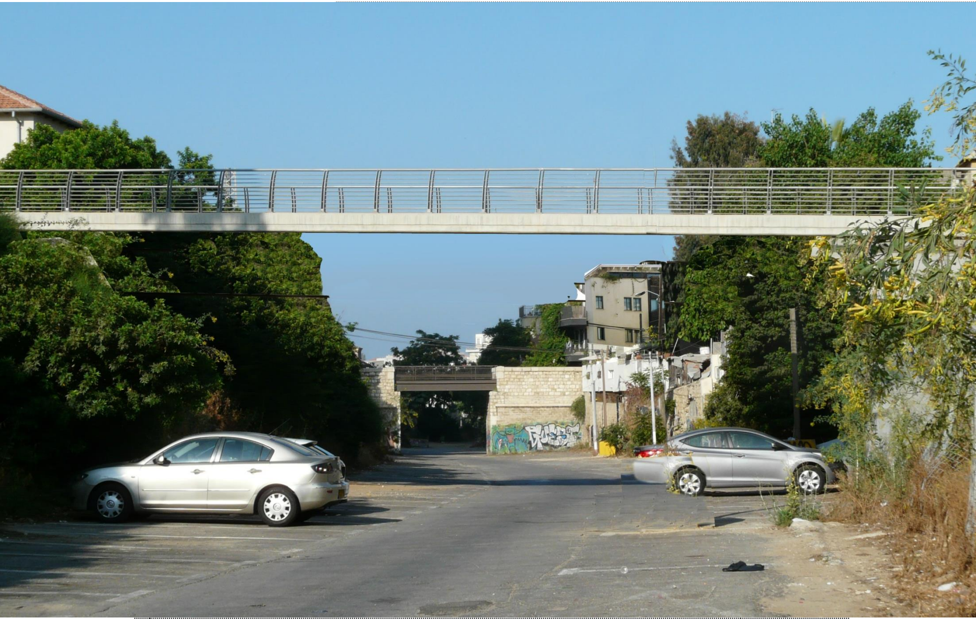
Nechushtan Bridge Tel Aviv
